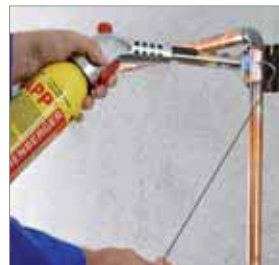
Hard soldering in gas installation
