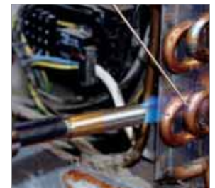
Hard soldering in refrigeration and climate control
