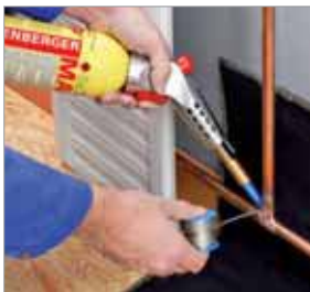
Soft soldering in heating installation
