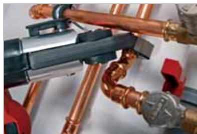
Working in confined spaces
