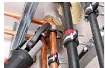
Working in confined spaces
