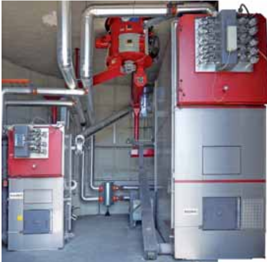
HPKI-W 300-1600 kW Forward feed series water-cooled
