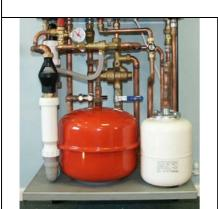
Fit the expansion vessel mounting plate (EVMP) to the frame (not shown in this picture). To do this, remove the lower two bolts holding the valve plate. Insert mounting plate and refit the two bolts to hold both the valve plate and EVPM in position.
