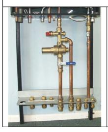
Open Bag 2 with two pipes. The 22mm pipe is for the gas, and the 15mm pipe for the towel rail return connection.
