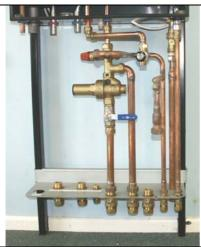
From Bag 1 take the 15mm pipe assembly with the thermostatic mixing valve. Assemble the pipework from the cold water manifold 15mm port, and connect to the 15mm hot water return valve on the valve plate. Loosely tighten joints.
