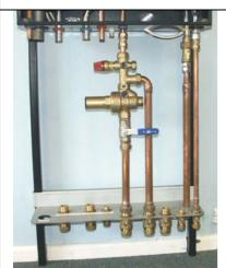
The auxiliary or towel rail connection is blanked off on the boiler with a hexagonal chrome plug. If this option is required, take the 15mm pipe from Bag 2 with a 15mm x ½" bsp male threaded compression fitting and a union. Remove the chrome plug (take care as residual water sometimes dribbles out) and fit the compression fitting. Connect to the towel rail flow union on the valve plate. If this is not required, simply discard the pipe or use elsewhere.
