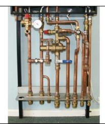
Fit the 22mm flow pipe using the 22mm compression connector at the boiler, and the union to the Valve plate. Remember the washer!
