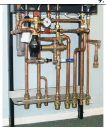
Take the 15mm safety discharge pipe with one bend, and connect to the 6 bar cold water pressure relief valve at the back of the boiler. Ensure that the pipe is fully inserted into the valve port, so that the compression olive grips the pipe.
