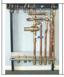
Fit the longer 22mm hot water outlet pipe from the 15mm port M to the hot water out valve on the valve plate. Don't forget the washer.
